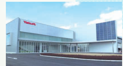
Solar panels at the Hyogo Miki Plant
