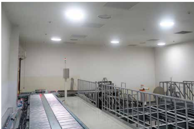
Solar lights at the Vietnam Plant (Yakult Vietnam Co., Ltd.)
