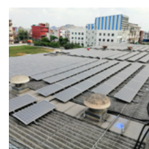
Solar panel installation
